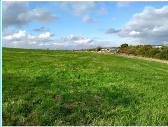
Location of the SMR facility, with the site being marked out with flags by the project team
